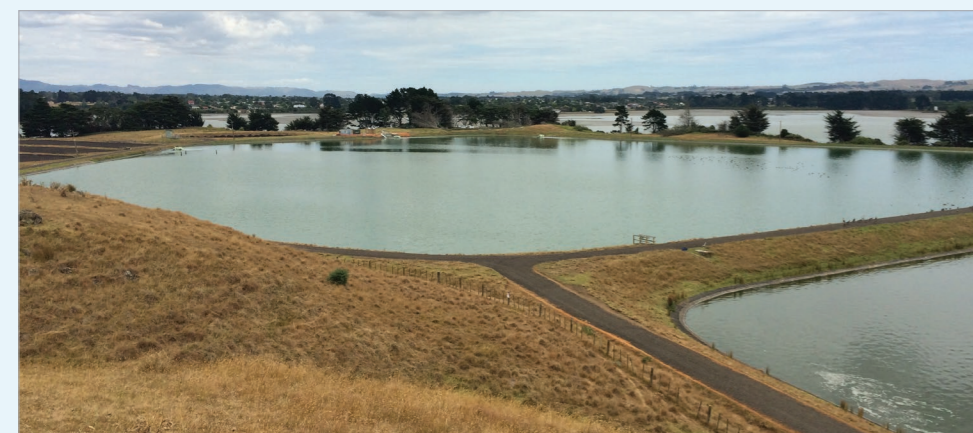
Waiuku Wastewater Treatment Plant.
